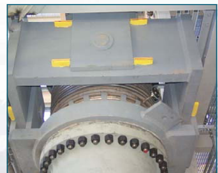
36" Gimbal Expansion Joint, designed for 680 PSIG and 540 °F, installed at chemical plant
