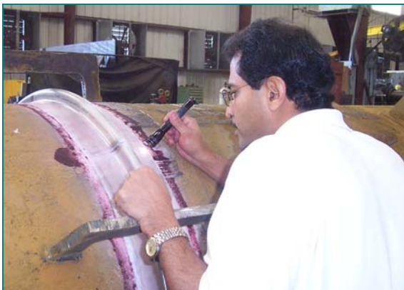
Dye penetrant test on the bellow's attachment weld of a 40" I.D. Single Coded Clamshell Expansion Joint
